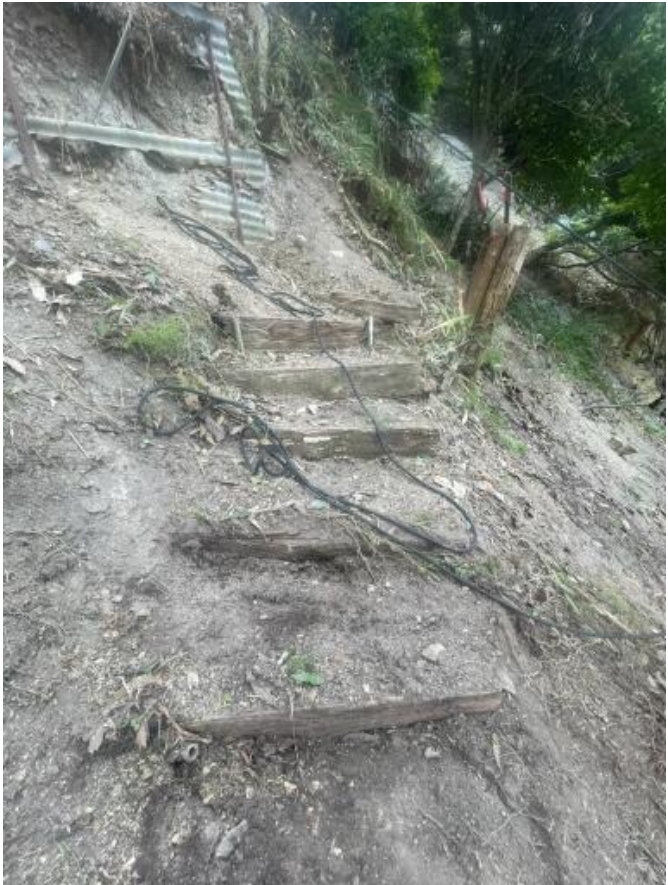
DECEMBER 2023 - EXISTING STAIR AND PATHWAY ADJACENT TO 217 BEACH ROAD.
