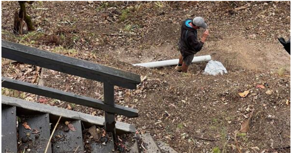
DECEMBER 2023 - STAIR FROM NEIGHBOURING BLOCK 217 BEACH ROAD TO RIGHT OF WAY.
